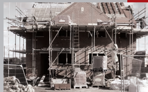
SMALL BUILDING SITES
